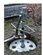
In addition to elevated pile loads, the paXos RFS can also be used for **building loads (BL)**, e.g. to base containers or prefabricated buildings. In this case, a special attachment distributes the weight load ideally over the precast concrete slab, allowing up to **16 tons of load** per foundation slab to be absorbed.
